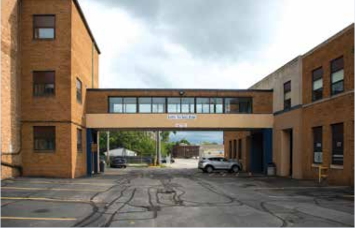
Current Exterior - North (Looking South)
